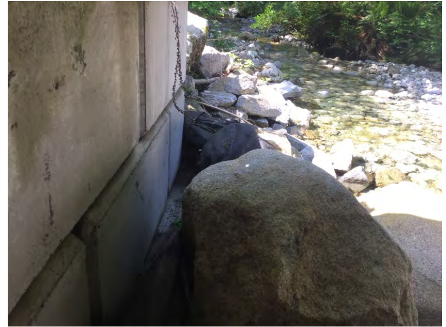
Downstream left bank spread footing visible
