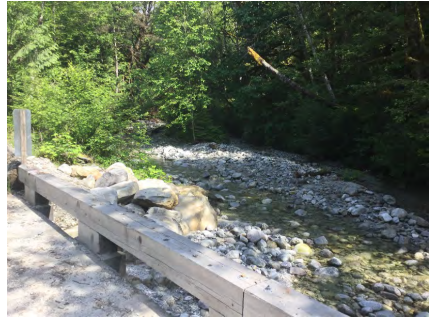
Upstream from Crossing
