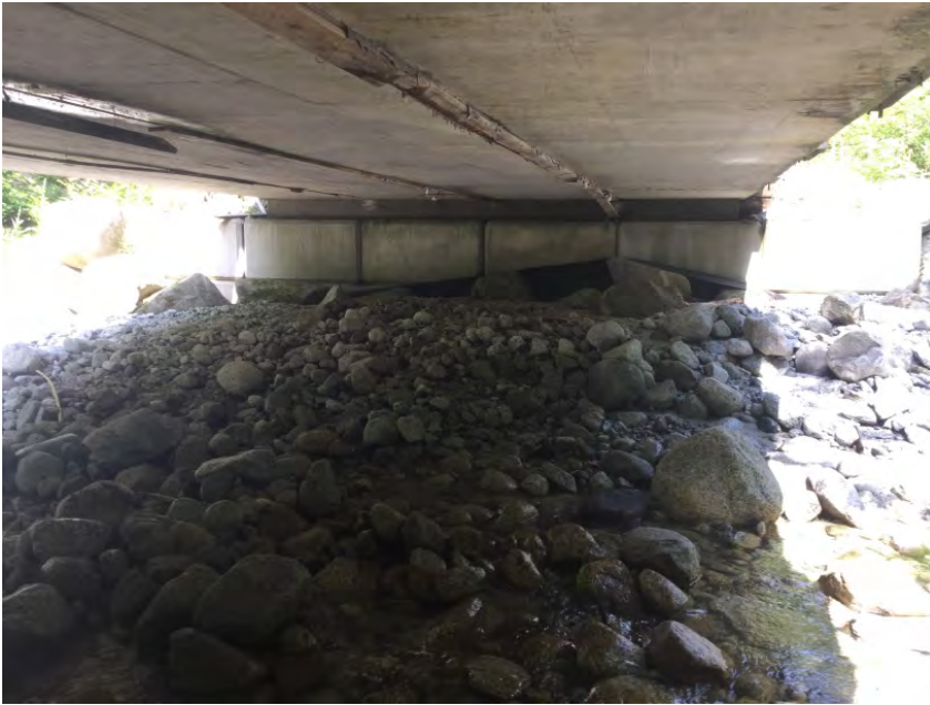
Right Bank Abutment when facing downstream
