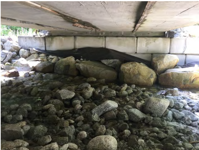
Left Bank Abutment when facing downstream
